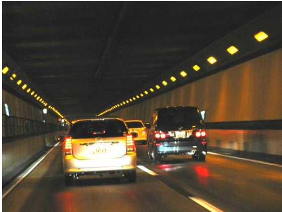
Ceiling panels of tunnel
