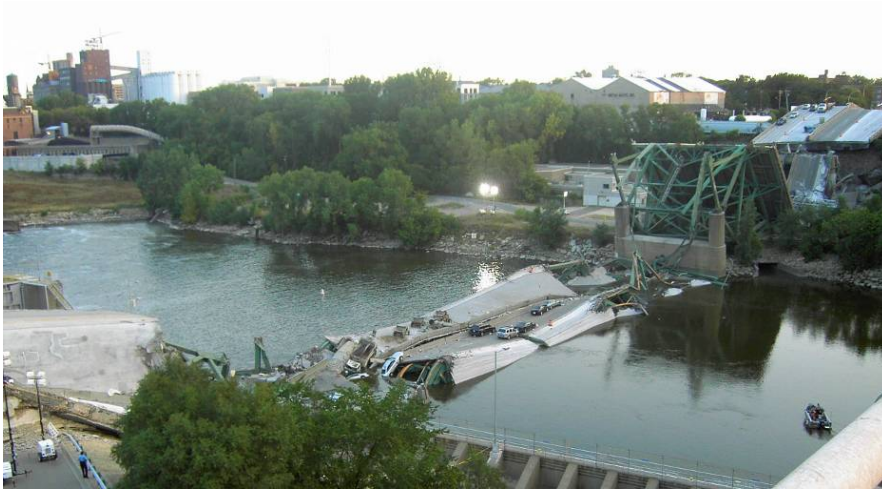
Collapsed I-35W Mississippi River bridge
