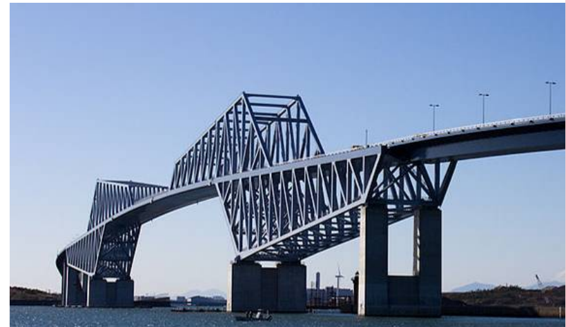
Tokyo Gate Bridge
