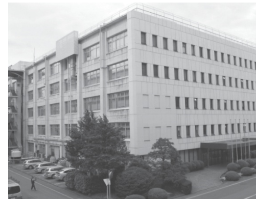
Building with installed vibration sensors
