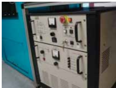
Figure 2. Typical YAG power station with DI water supply.
