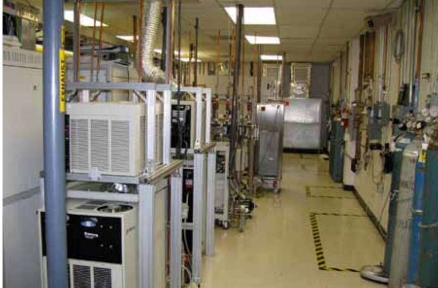
A portion of ALLVIA's TSV fabrication equipment farm.
