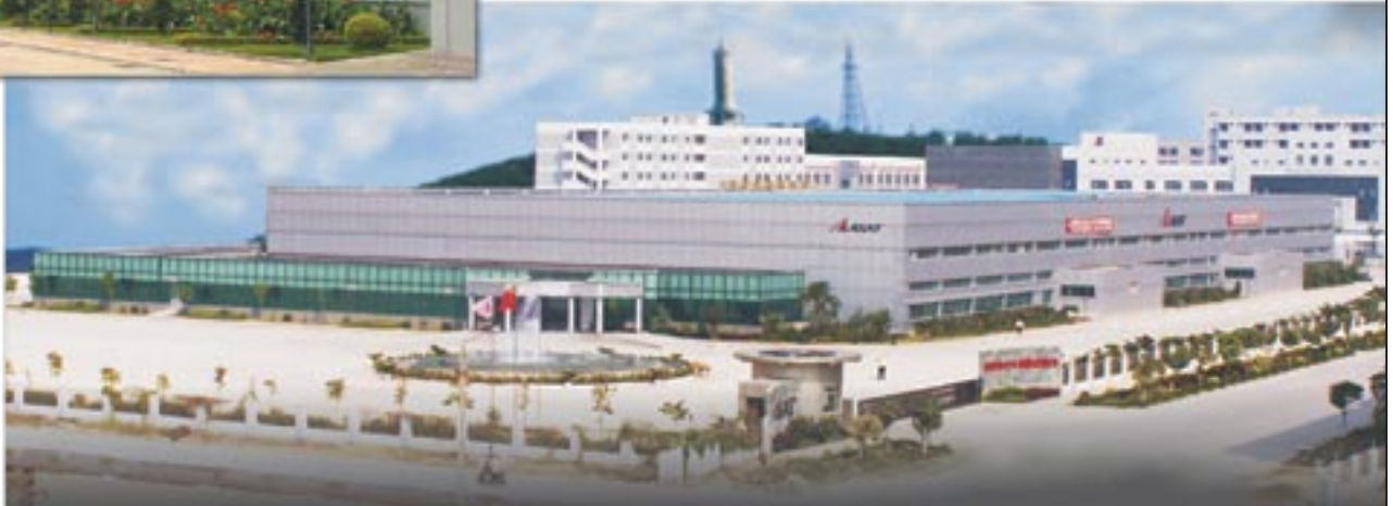
Phase 1 of ASAT's new state-of-the-art manufacturing facility in Dongguan, China.
