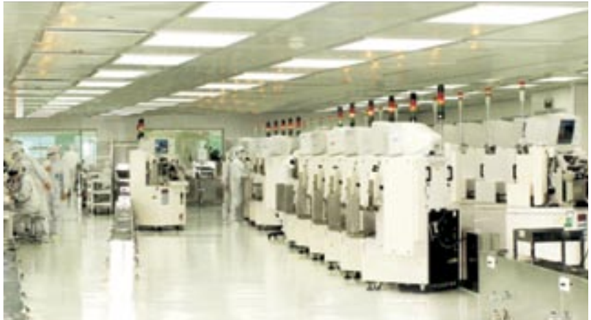
Clean-room in Phase 1 of ASAT's China facility.
