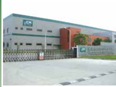
Factory #2 - Hefei Economic & Technological Development Zone, Hefei, Anhui Province
