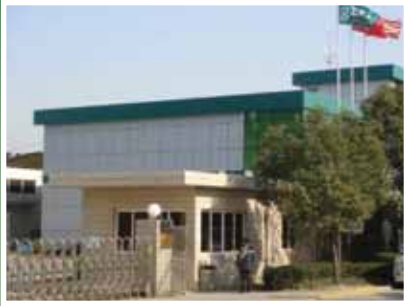
Founding Factory #1 - Jiading Industrial Development Park, Shanghai, China
